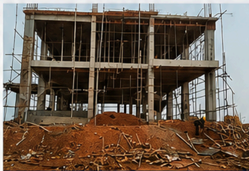
STRUCTURE IN PROGRESS
