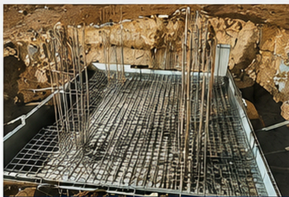
RCC FOUNDATION WORK
